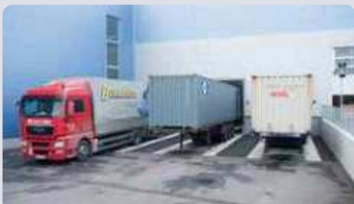
Daily incoming and outgoing goods
